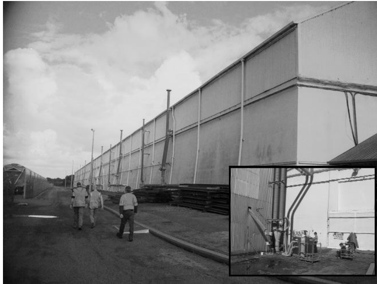
Fig. 3- The 300,000 ton capacity sealed horizontal shed at CBH Kwinana Grain Terminal Western Australia with insert HDS 800/VAPORPH 3 OS fumigation setup.
