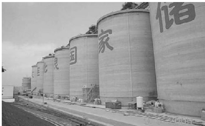
Fig. 5- The on-site mixing of VAPORPH 3 OS ® with bulk CO 2 at Dalian Phase-2 silo block of 20 bins by 30,000 ton capacity each.
