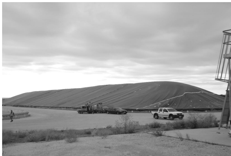
Fig. 4- A 20,000-ton bunker with the HDS 800/VAPORPH 3 OS fumigation setup at GrainCorp Nhill grain storage center in Victoria Australia.
